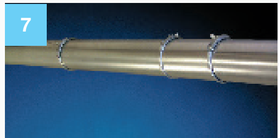
Finished connection with the slip duct.
