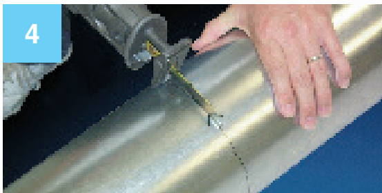
Cut the duct.
