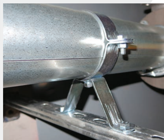
Duct mounted with Split Strap and Legs for Split Strap.
